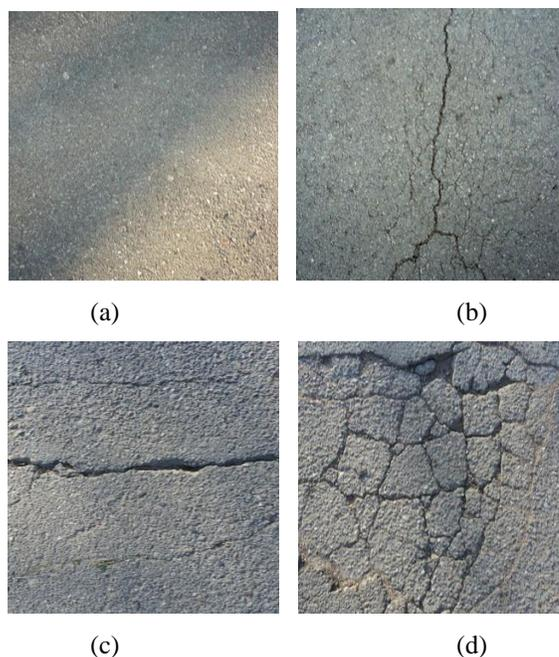
Fig. 1. Different types of road surface cracks; a) Healthy pavement without cracks, b) Transverse crack, c) Longitudinal crack, d) Mesh type crack
