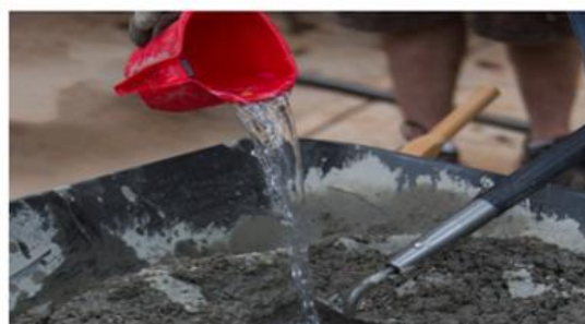
Fig. 6 Preparation of concrete mix with water
