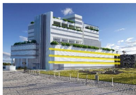
Figure 5.7. View of Kian Hospital
