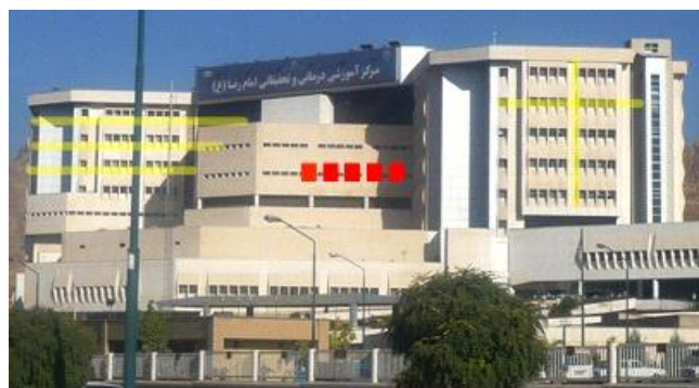
Figure 5.3. View of Imam Reza Kermanshah Hospital
